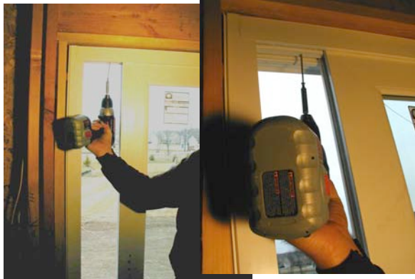
Screws are placed just above the door in the header, eliminating upward motion.
